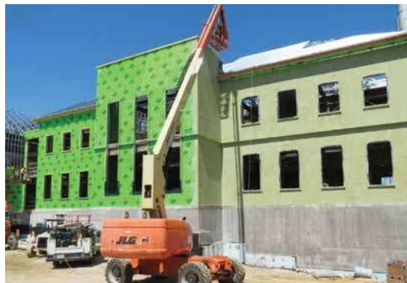
Vapor barrier installation with spray or roll-on
