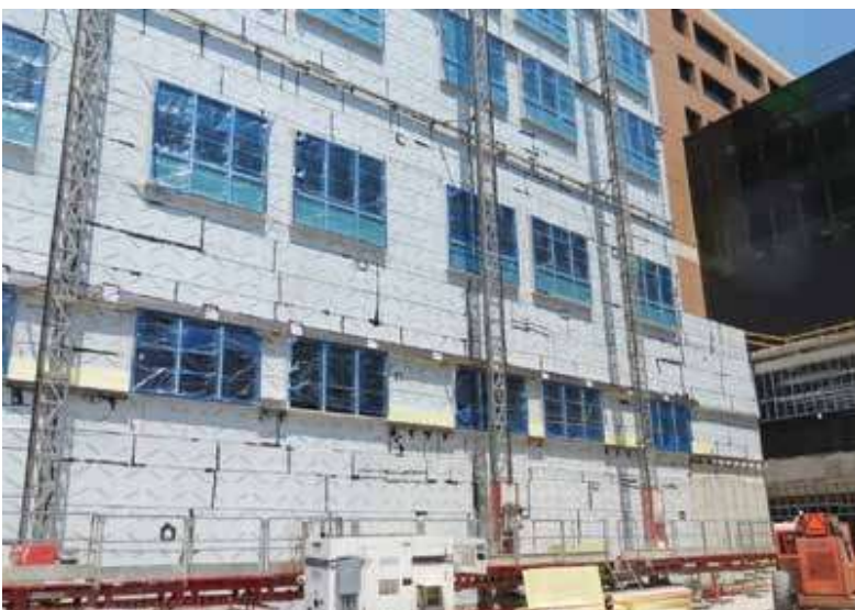
Vapor barrier installation with self-adhered sheets
